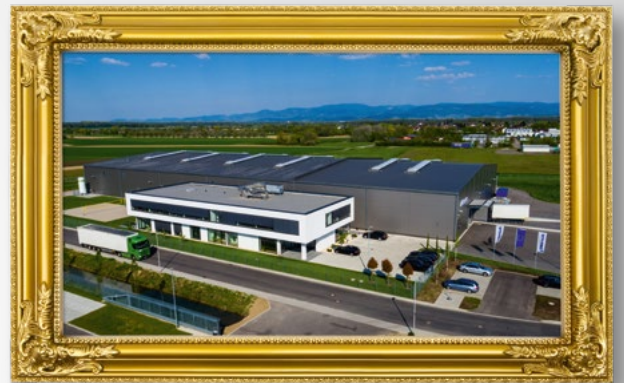
2017 New plant in Willstätt
